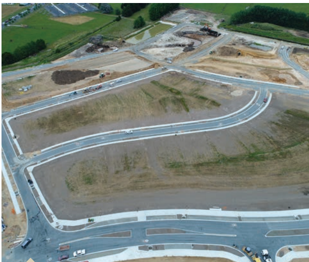
New streets start to take shape at Rotokauri
