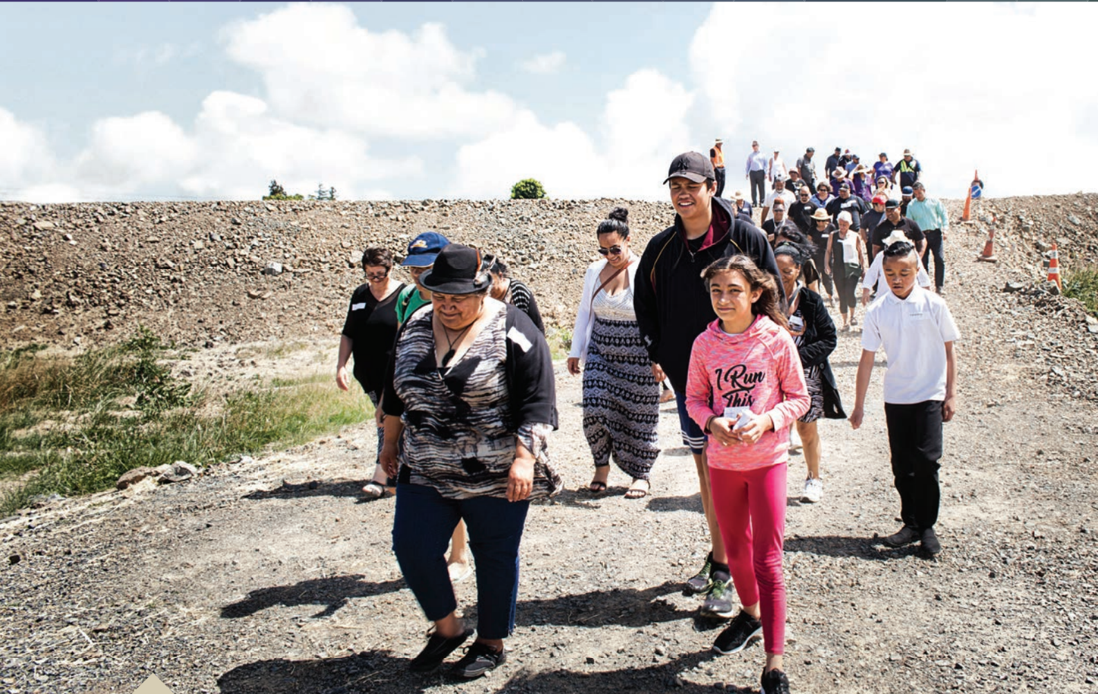
Kaimahi of Waikato-Tainui tour the earthworks for the inland port at Ruakura
